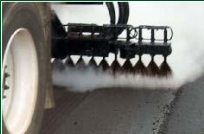
Proper Spraying - Even
